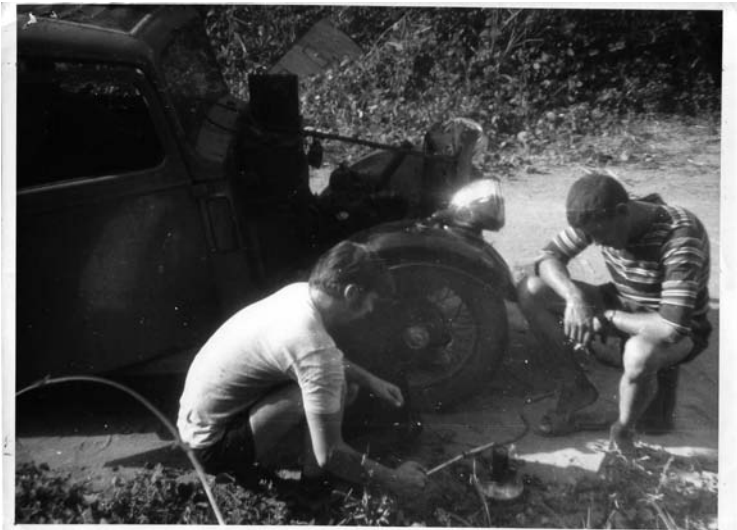
Congo February 3, 1969, on the way to Buta. Werner and Arthur using Primus stove to solder radiator.
